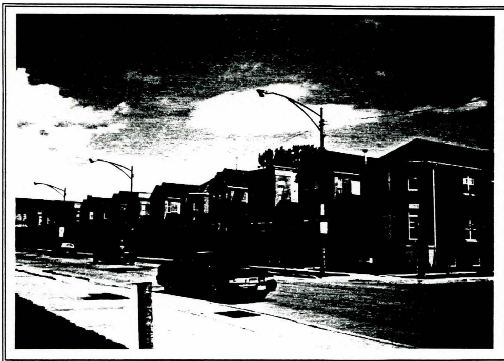
View of adjacent SFR section
