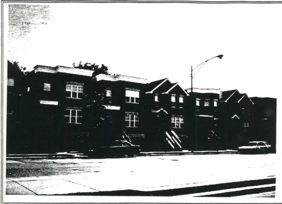
Front view, sample units
