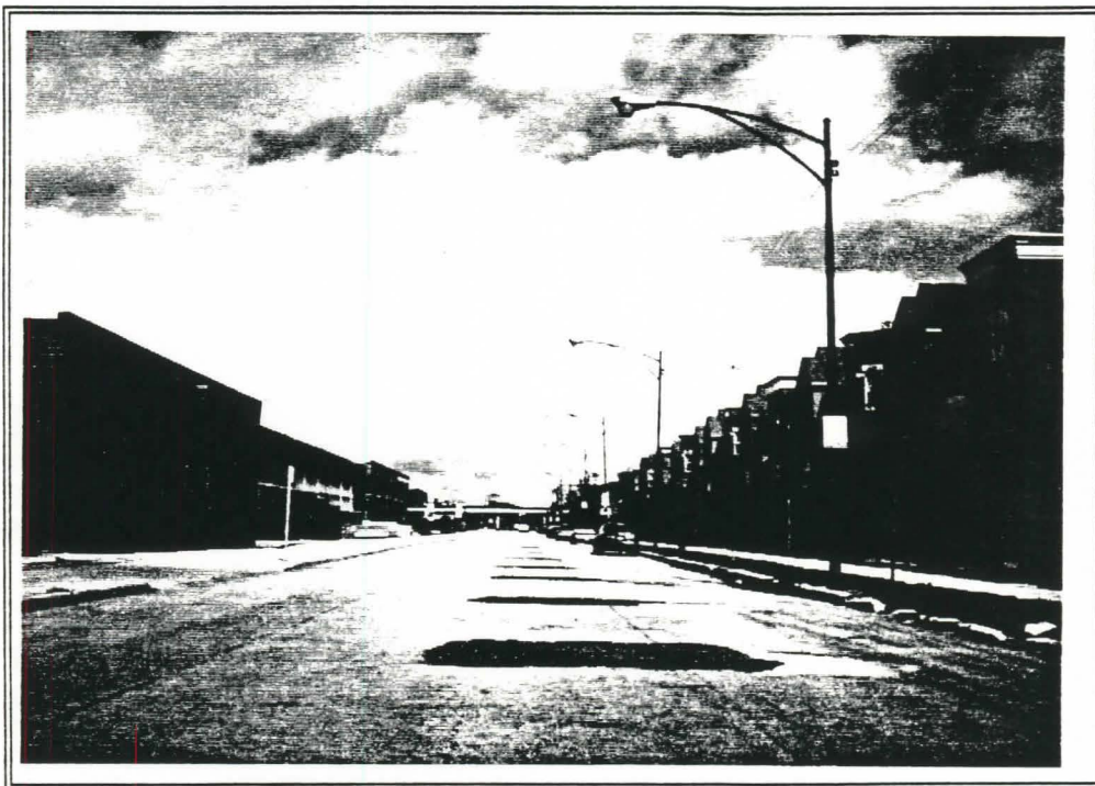
View northerly along Larrabee Avenue
