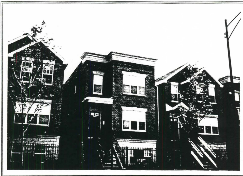
Front view, sample units
