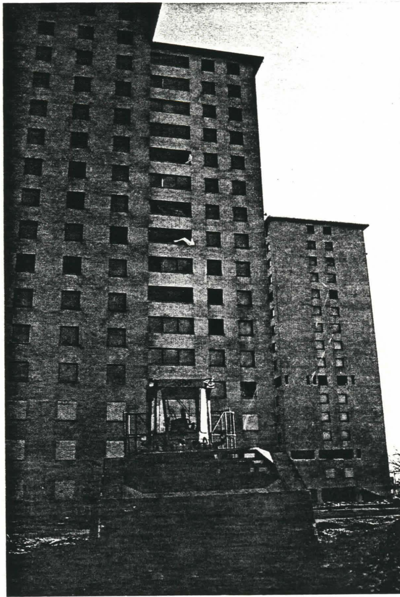
The building at 1130 East 41 st Street – North Elevation (In the background is the building at 4155 South Lake Park Street – North Elevation)
