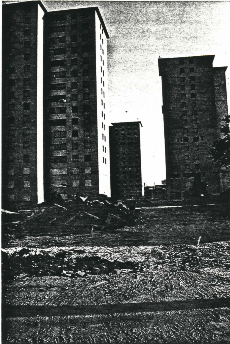
In the foreground is the building at 1130 East 41 st Street – North Elevation In the center (and the rear) is the building at 1132 East 42 nd Street – North Elevation On the far right is the building at 4155 South Lake Park Street – North Elevation
