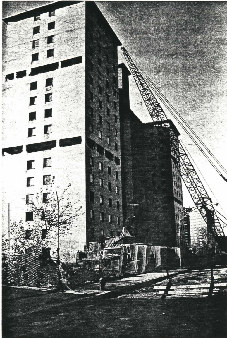
The building at 4040 South Oakenwald – East Elevation (South Elevation in sunlight)
